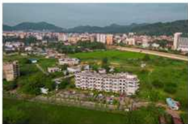
Aerial View of Our Campus
