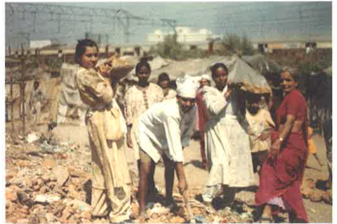
The Umang group helping to build a member's house.
