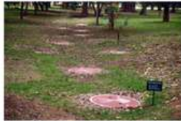
Field example of Recharge/ Percolator pits (Lalbag, Bangalore)
